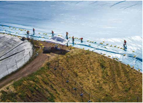
The workers were dwarfed by the massive dam cover being installed at Oonooie. They completed the job just before the weather closed in
