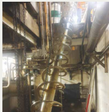
The old screw conveyor being removed
