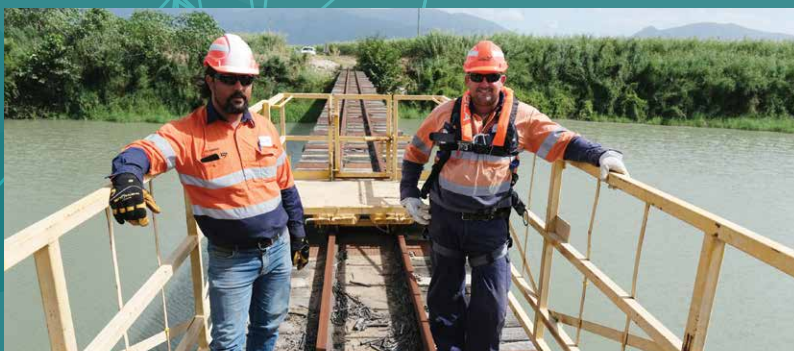
Civil Supervisor Lee Fabbro and Senior Civil Coordinator Jared Hervey helped to reinstate the spans of the Haughton cane rail bridge at Giru. Three spans are removed each year ahead of the wet season to reduce the risk of the bridge being damaged during flooding of the Haughton River.
