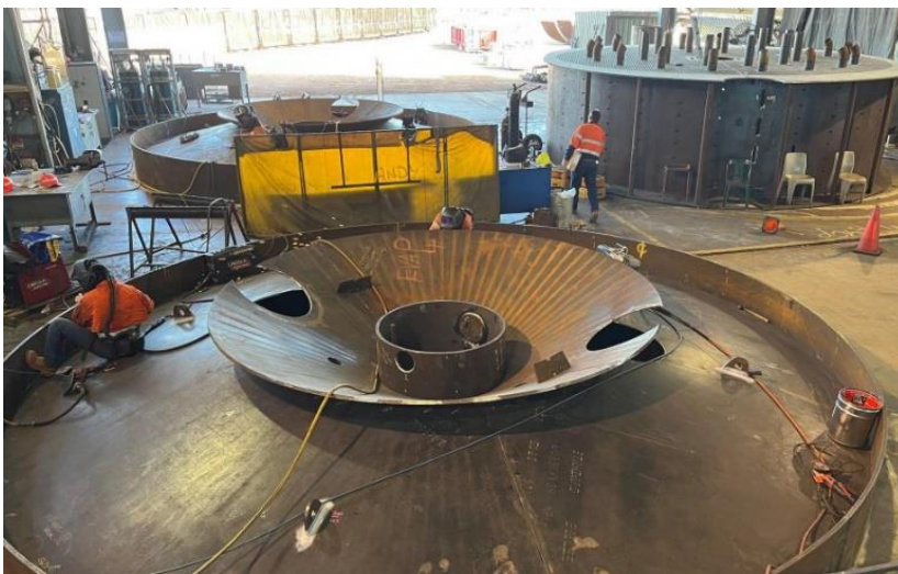
Project work is on track for the two evaporators being built in-house at Wilmar Sugar's workshops ahead of the 2023 season.
