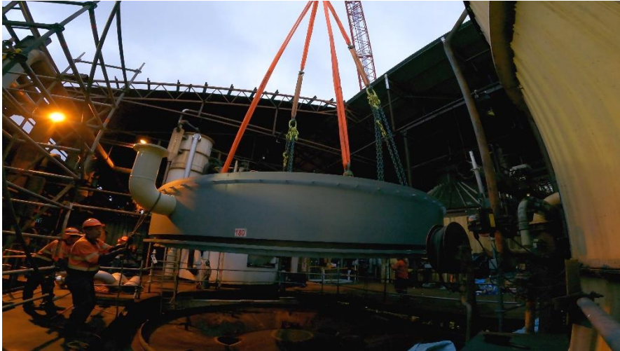
Wilmar's Proserpine Mill employees guide the calandria into position.
