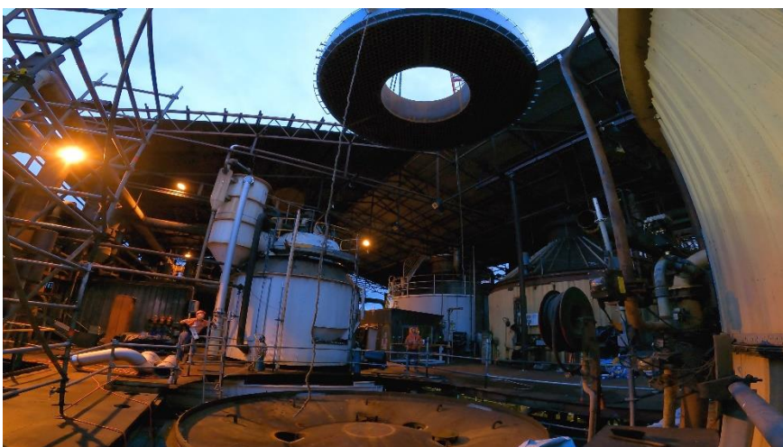
The 37-tonne calandria is lowered into the factory.
