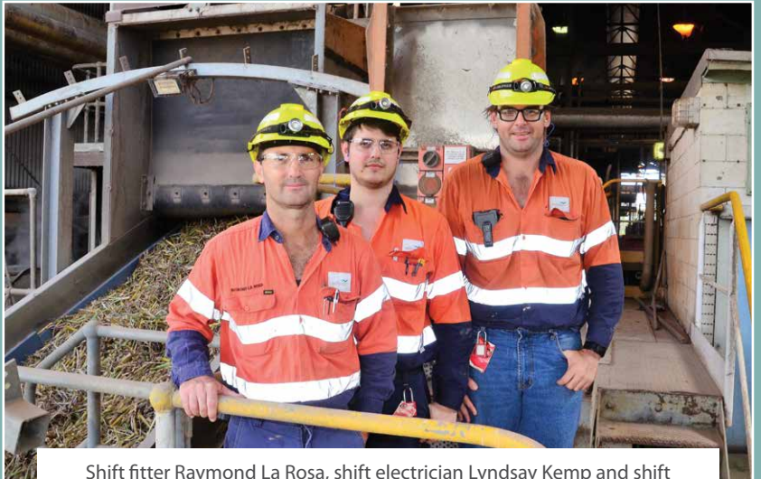
Shift fitter Raymond La Rosa, shift electrician Lyndsay Kemp and shift coordinator Daniel Castorina witness some of the last cane for the season head towards the A-side shredder at Victoria Mill.
